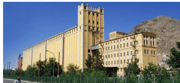
Reactivation of Silos
