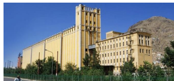
Reactivation of Silos
